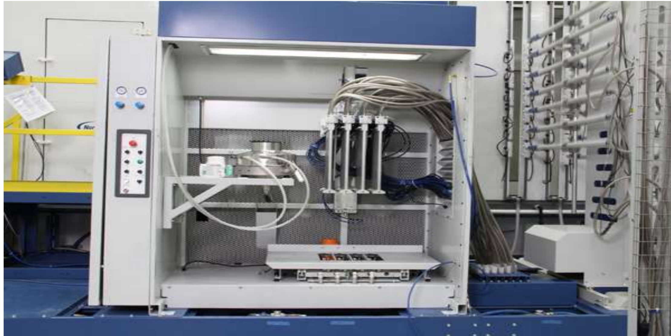
Feed Center with internal gun purge and 14" sieve.
